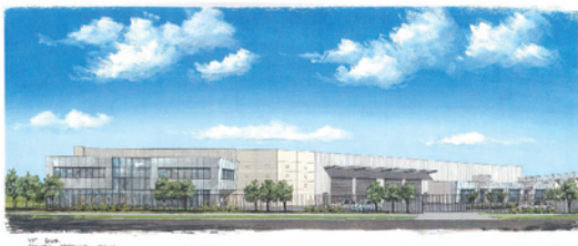
UNITS 1-3 17 AIRPARK DRIVE AIRPORT OAKS
